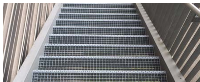
Treads for straight stair
